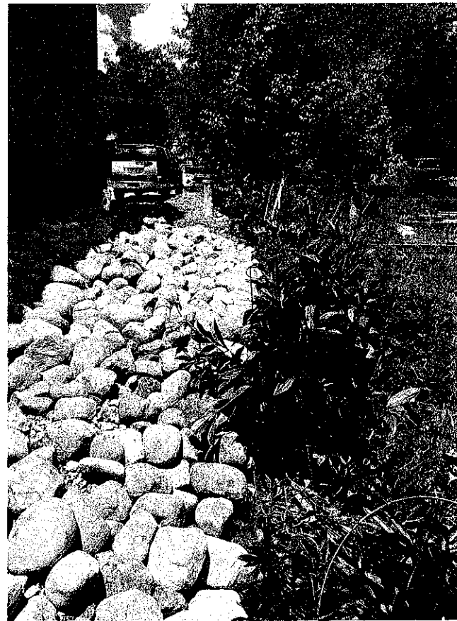
LEFT ELEVATION ROCK DITCH
