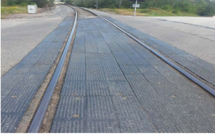
Figure 4 - Rubber Crossing Surface
