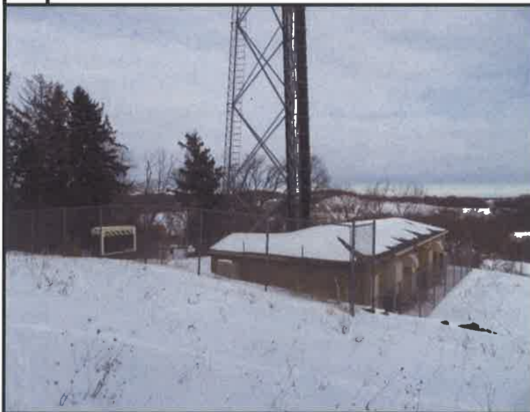
B COMPOUND OVERVIEW
