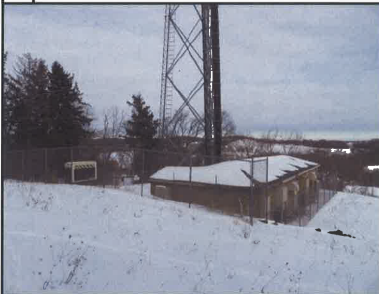
B COMPOUND OVERVIEW
