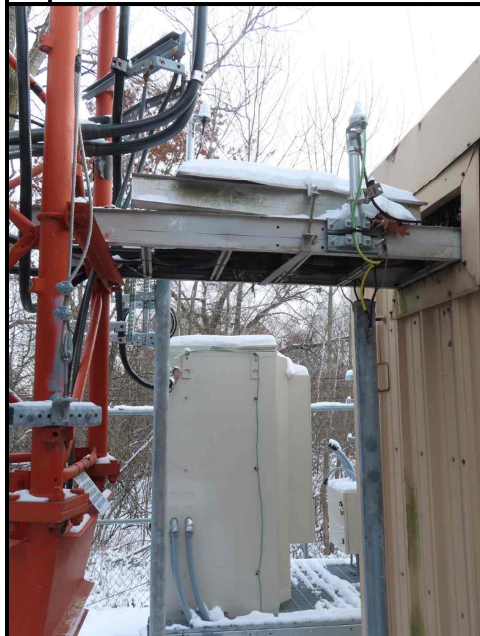
E ICE BRIDGE HANGER
