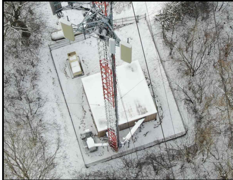
B COMPOUND OVERVIEW
