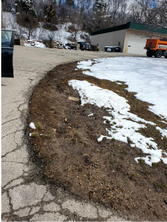
Erosion Area of Concern
